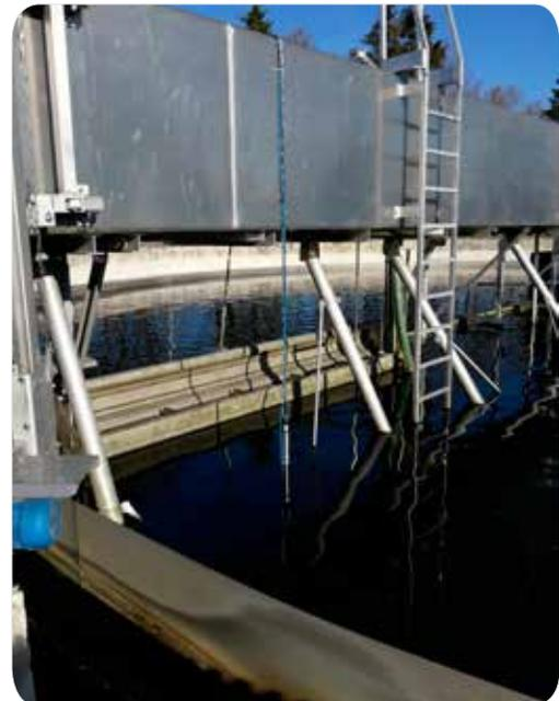
Fig. 1-2: Installation of the NiCaVis® 705 IQ sensor in the clarifier of the wastewater treatment plant Peißenberg
